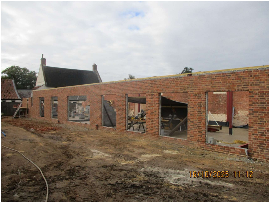
Evidence of retained bricks
